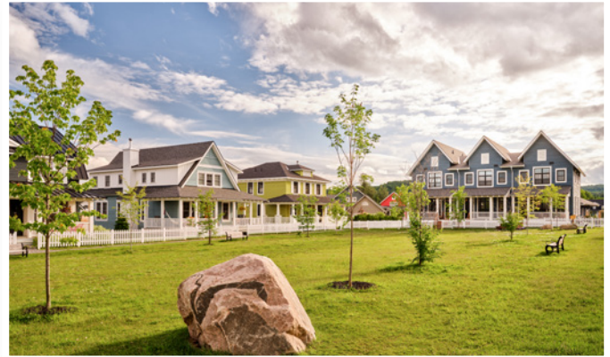
Townhomes at Landlab's Hendrick Farm project
