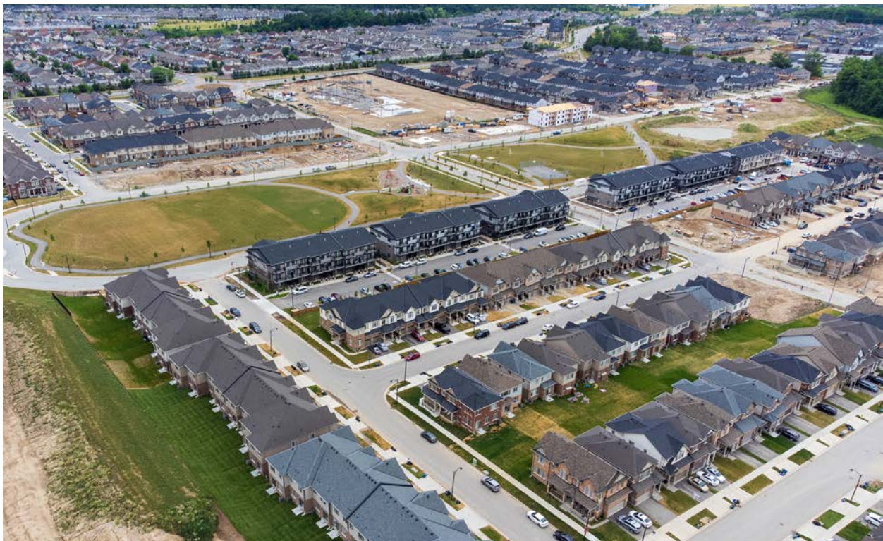
Figure 8: Construction at Schlegel's Wallaceeton community. A full range of housing including detached forms and street and stacked townhomes are under construction along with a new elementary school.
