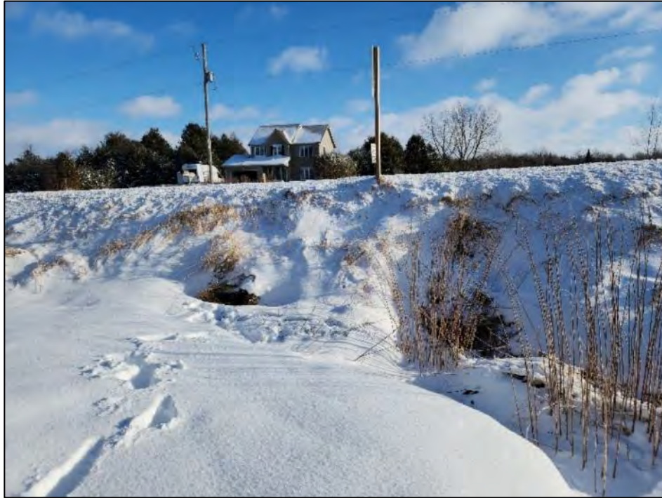
Photo 11. Twinned inflow culverts in the northeast corner of the property (December 21, 2022).
