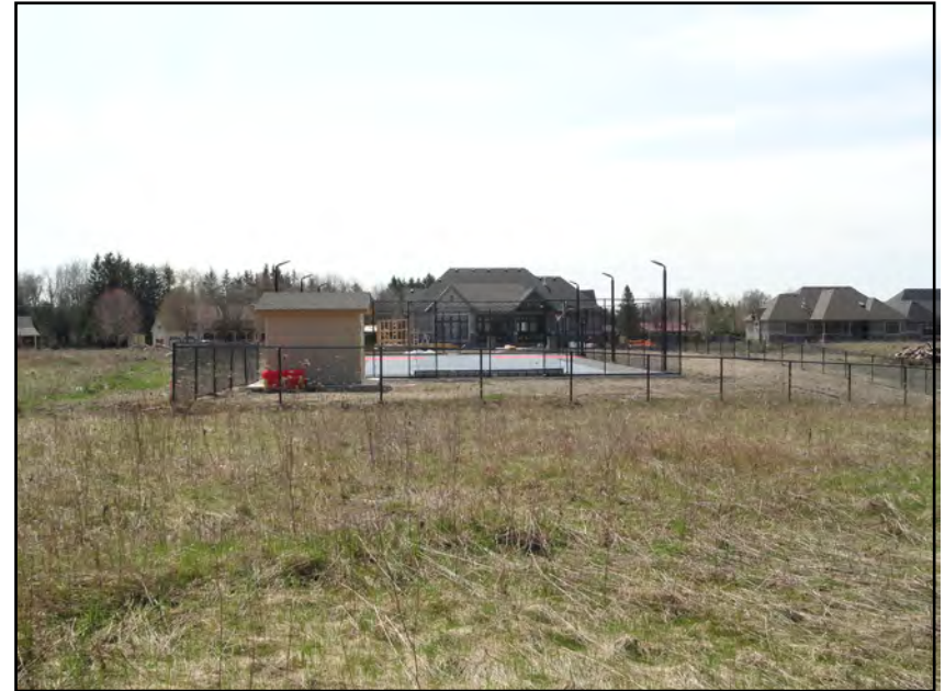
Photograph 2. Southward view of an existing estate lot under construction, along north side of Ormiston Street, abutting the south side of the subject property
