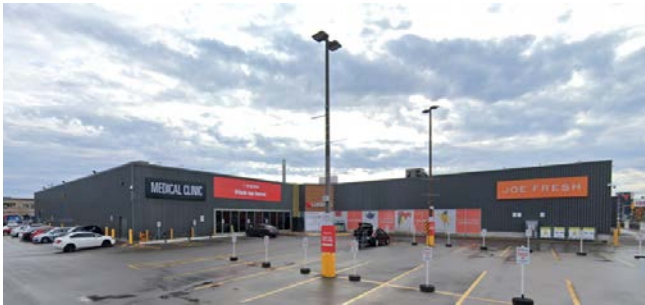
Subject Site from Eastern Avenue
