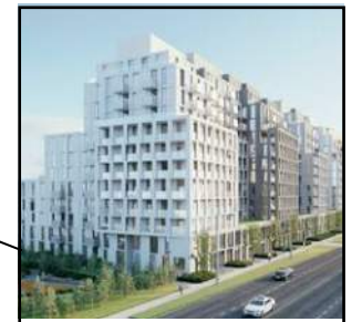
530 Wilson Ave Construction 12 Storeys
