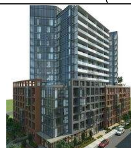
4-6 Tippett Rd Construction 16 Storeys
