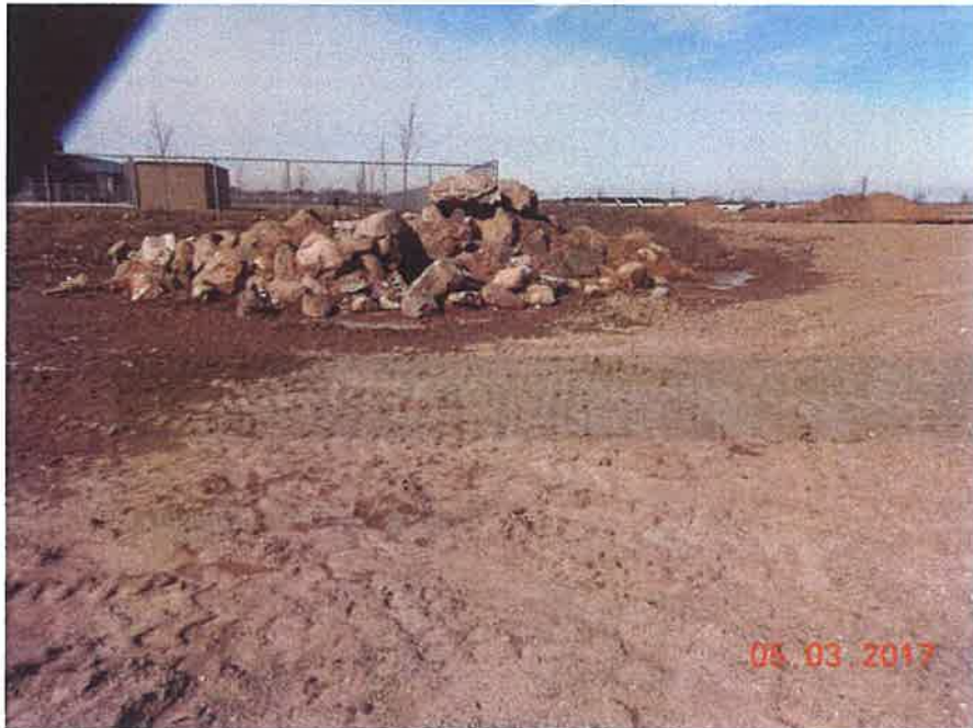
Photo 2 – looking west toward along back fence of the elementary school
