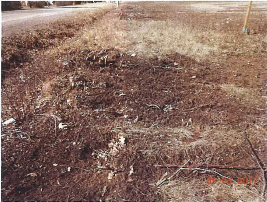
Photo 5 – looking west along Barton Street
