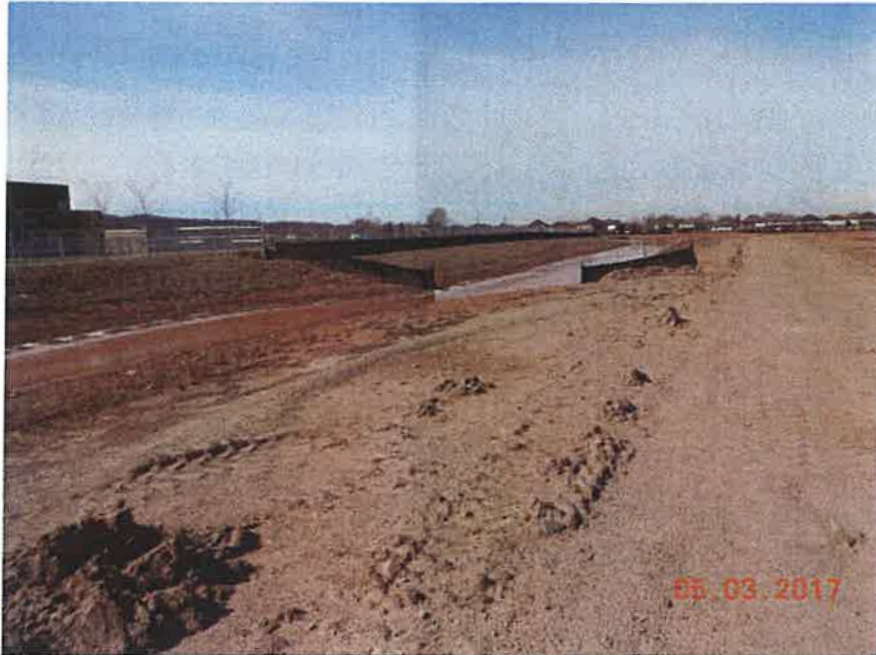
Photo 3 – looking west - large ditch behind elementary school
