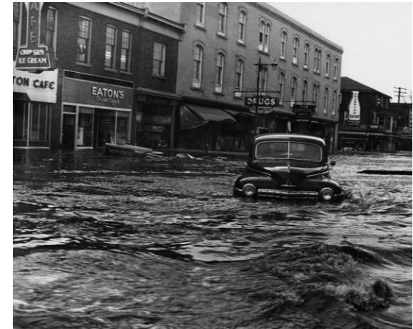
Main Street North after Hurricane Hazel, March 1948. Russell Cooper fonds, Region of Peel Archives/PAMA
