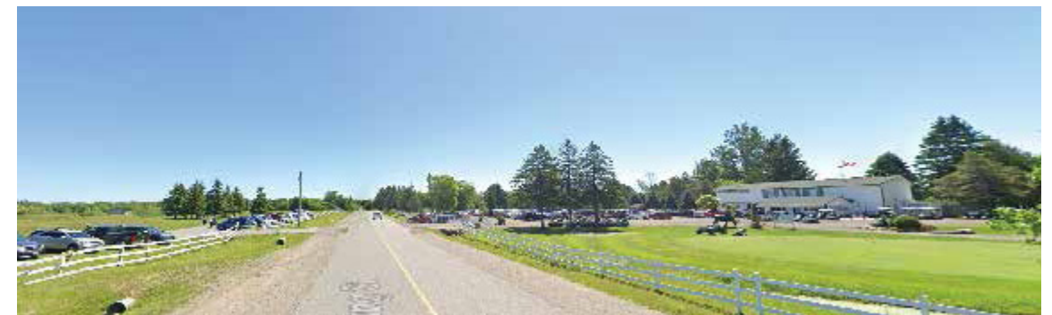
VIEW ALONG KING STREET LOOKING EAST
