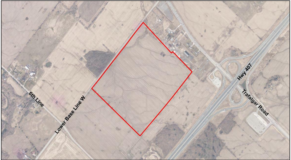
Figure 1 – Air Photo of 0 East Lower Baseline, Milton
