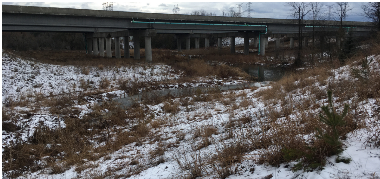
Highway 407 span bridge, Oshawa Creek, Oshawa, ON
