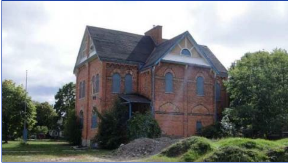
Figure 9: Connaught Public School Before Restoration 19
