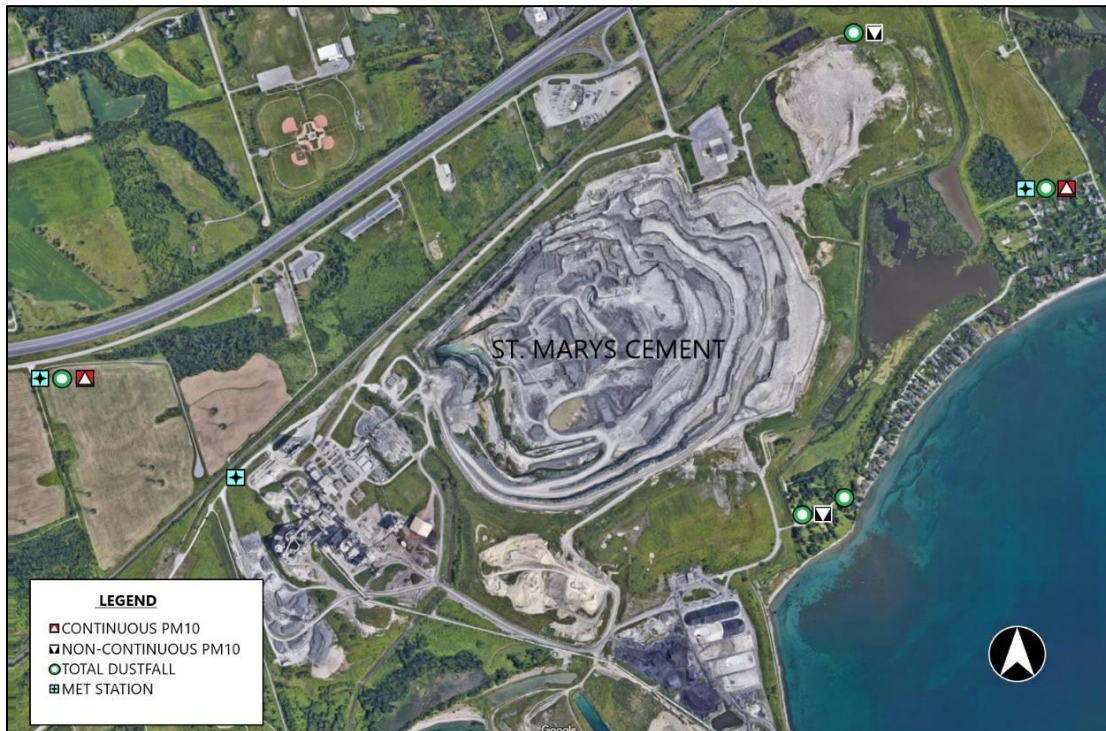
Photo 2: St. Marys Bowmanville Cement Plant PM Monitoring network (modified Google Image, 2020)
