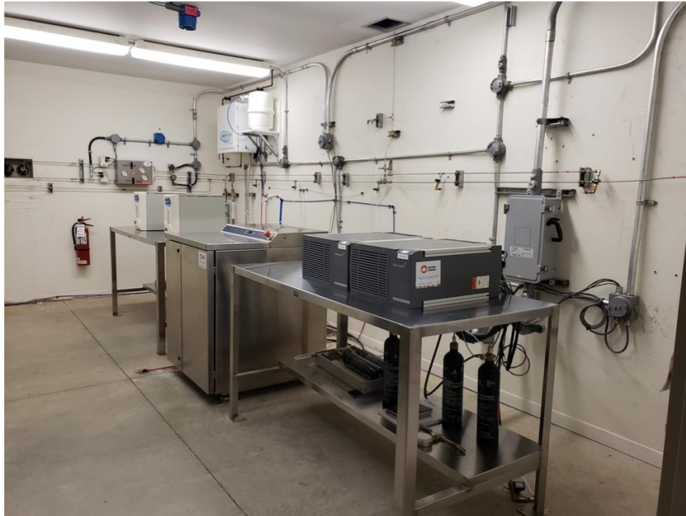
Figure 2. Two views of Hydrogen Lab with 3 electrolyzers and 5 fuel cells and required piping to the storage facility outside of the building
