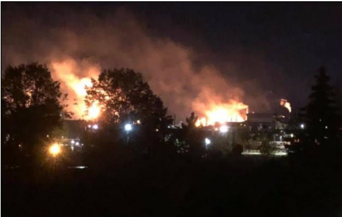
Heavy emissions and flaring from ASI on October 18, 2019 due to pipe bursting (Soo Today)
