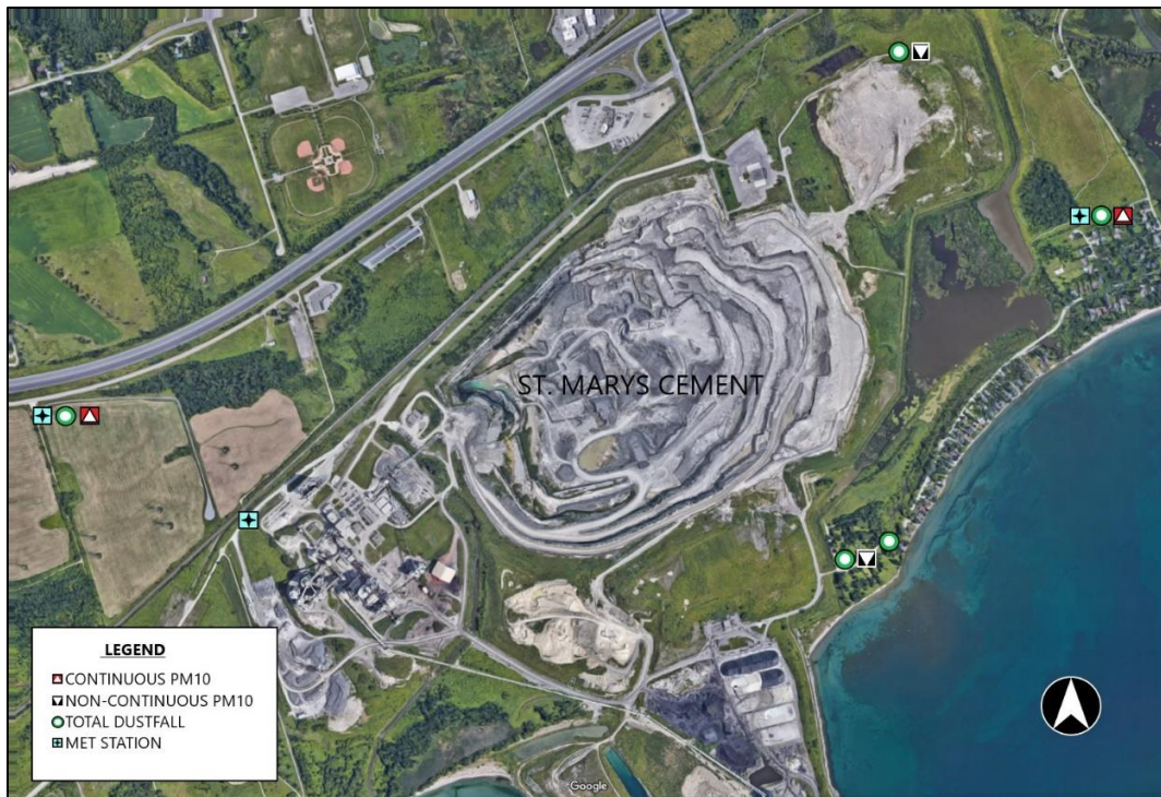
St. Marys Bowmanville Cement Plant PM Monitoring network (modified Google Image, 2020)
