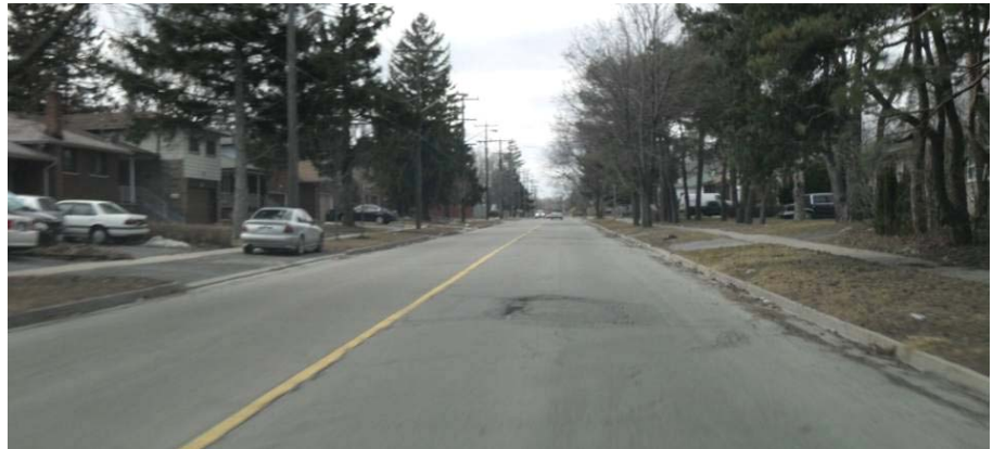
Figure 5. Pavement on Coronation Drive West of Manse Road
