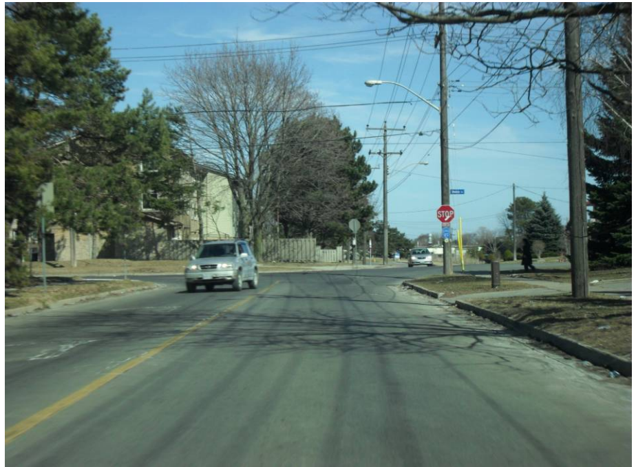
Figure 10. Offset Intersection of Coronation Drive at Manse Road
