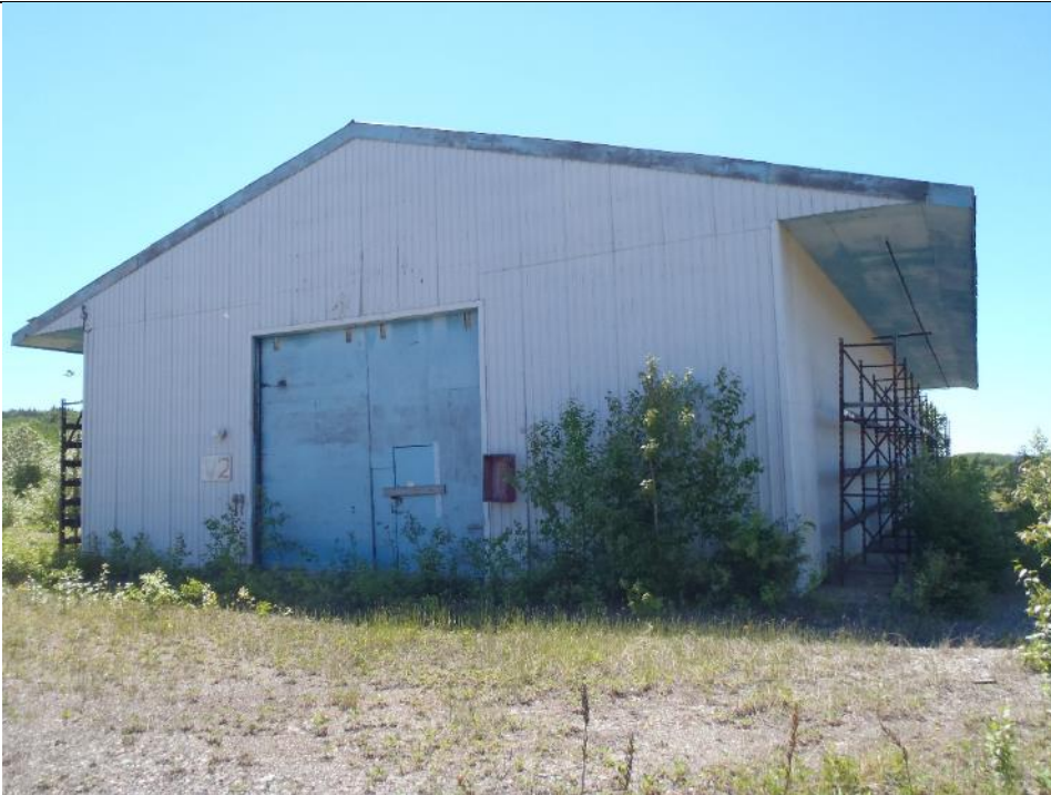
Photo 37: New cold storage building. Facing southeast.
