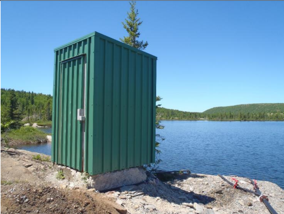
Photo 51: Moran Lake Pump House supplies water to the Water Treatment Plant. Facing west.
