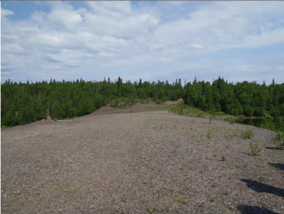
Photo 13: Upper Dam. Facing northwest.
