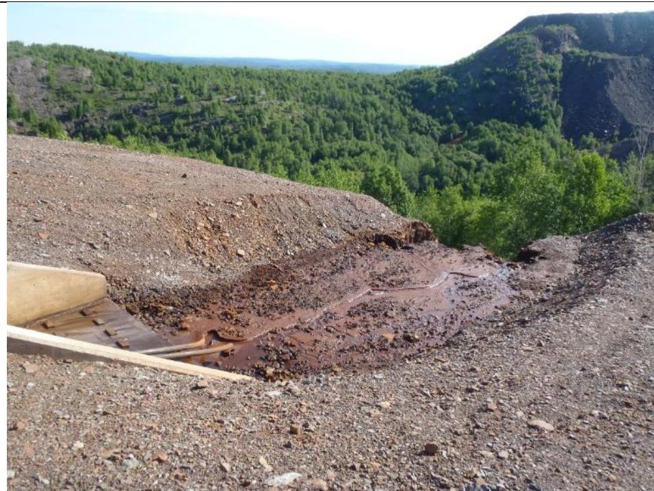
Photo 30: Drain from clarifier to Boyer Lake. Facing north.
