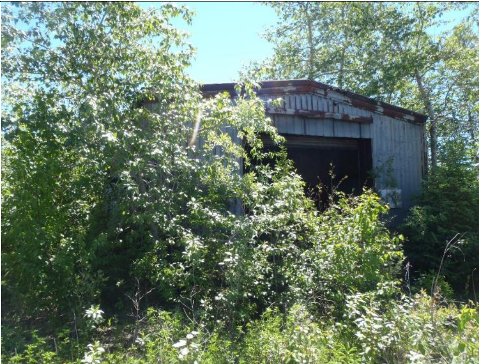
Photo 52: Motor Storage Shed. Facing east.
