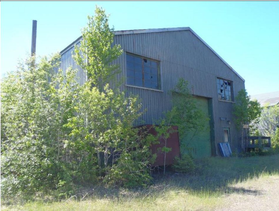
Photo 48: Machine Shop, back of building. Facing south.
