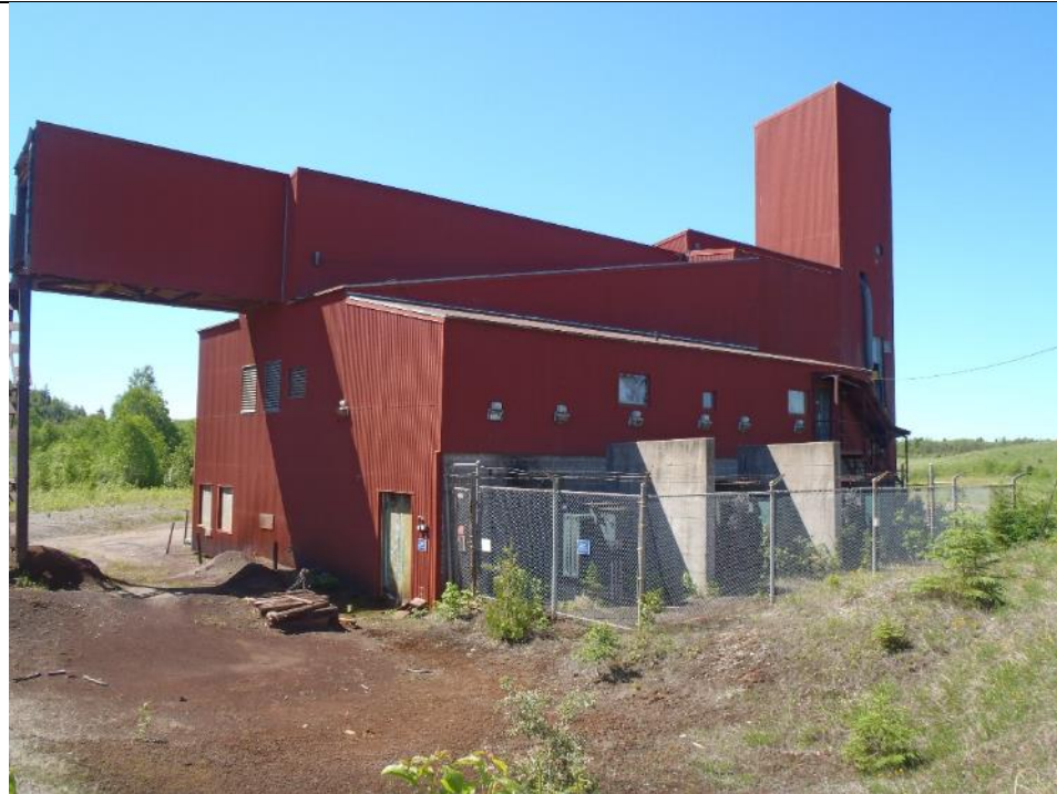
Photo 77: Three transformers on north side of the Cable Belt Drive House. Facing south.
