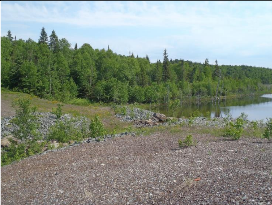
Photo 15: Upper Dam Spillway. Facing north.
