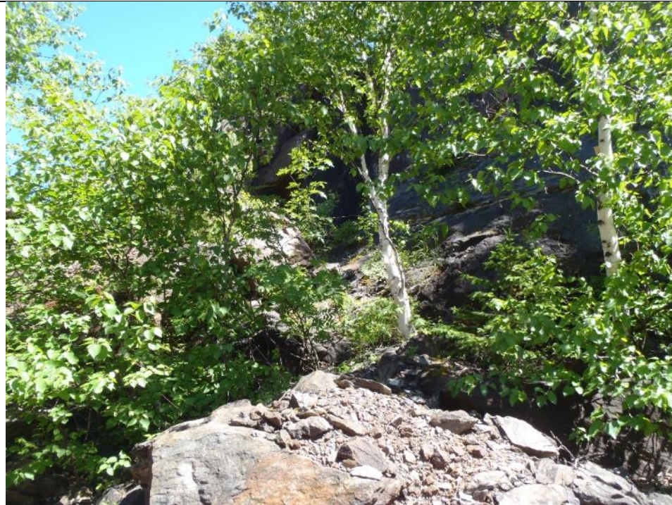
Photo 5: H-272 Exhaust Raise showing sloughing of pit walls. Facing north.
