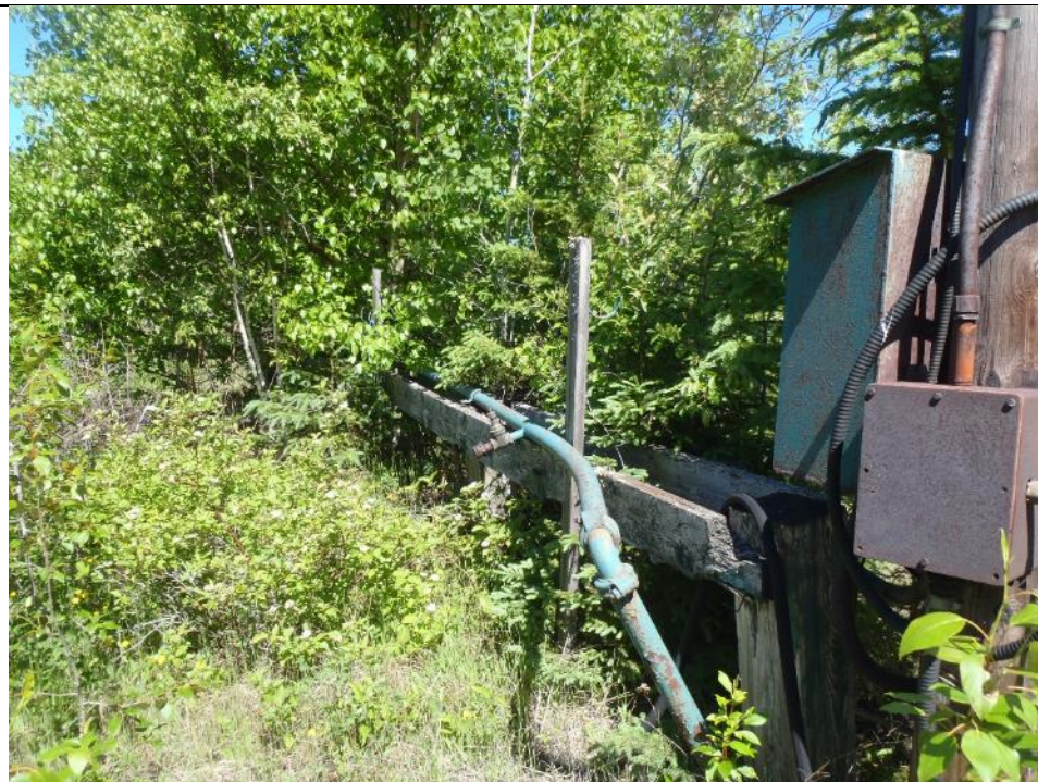
Photo 64: Trestle for water line. Facing northwest.
