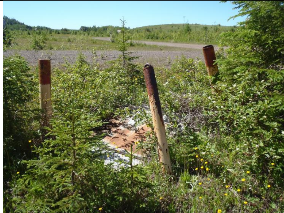
Photo 11: Drainage sump on Sinter Plant site. Facing south.
