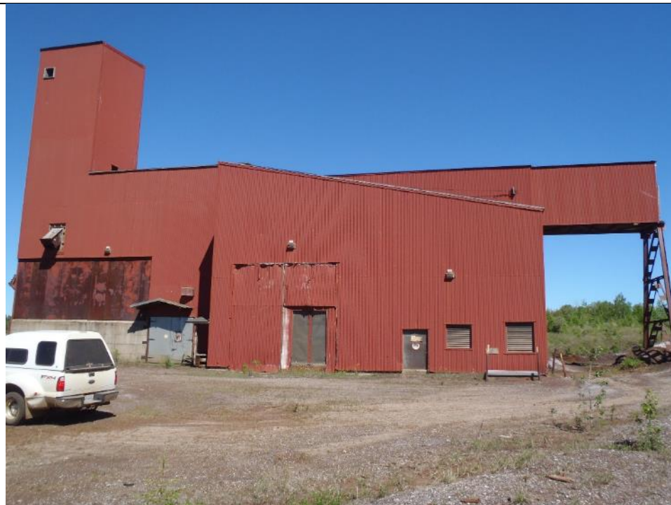
Photo 34: Cable Belt Drive House showing no significant changes. Facing northwest.
