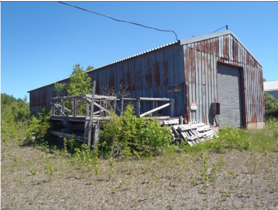
Photo 50: Metal Gold Storage. Facing northeast.
