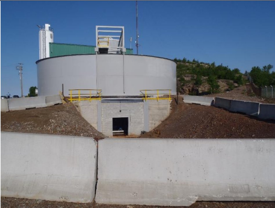
Photo 69: Water Treatment Plant Clarifier showing access. Facing northwest.
