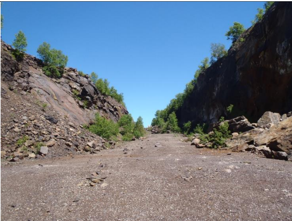
Photo 10: Victoria Pit showing increased sloughing from pit walls. Facing east.
