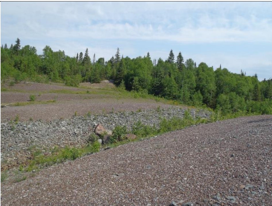
Photo 16: Upper Dam Spillway. Facing north.
