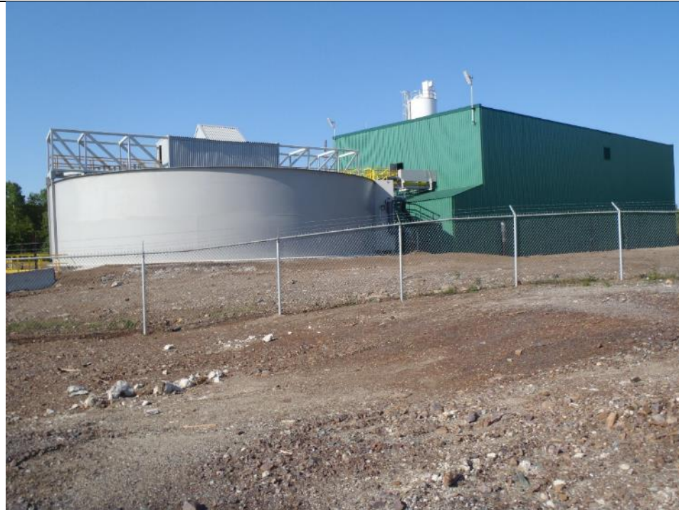
Photo 67: Water Treatment Plant and Clarifier, back view. Facing southwest.
