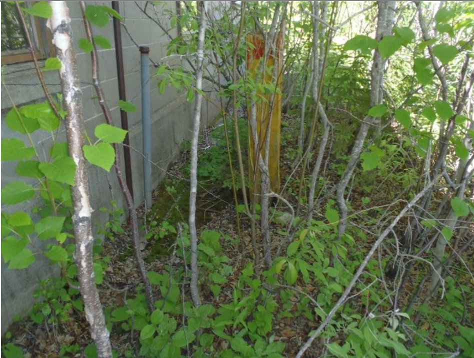
Photo 81: Two oil tanks are buried on the northeast side of the New Garage building. Facing northwest.
