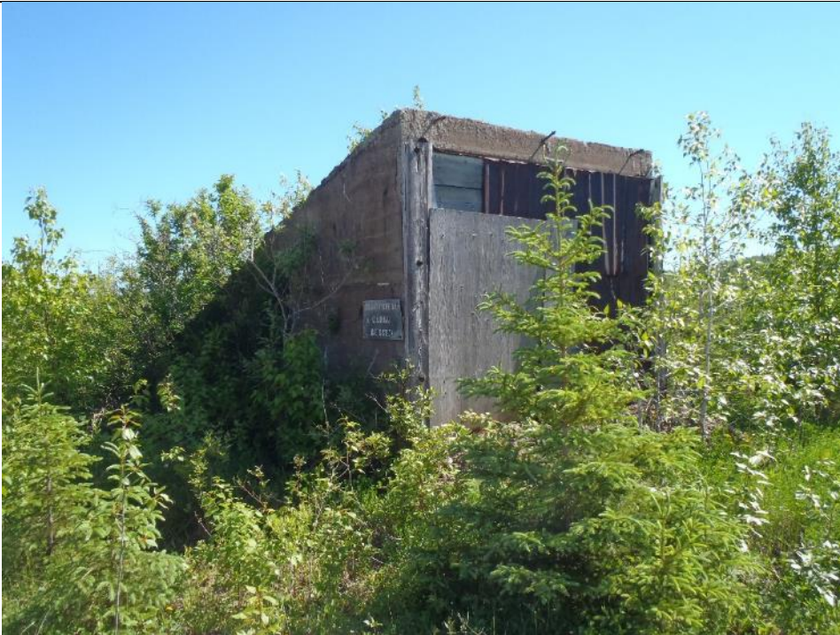
Photo 7: Entrance to Josephine Tunnel. Facing northeast.
