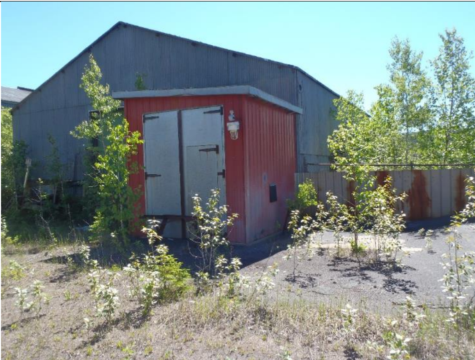
Photo 58: Pipe Shop, back. Facing east.
