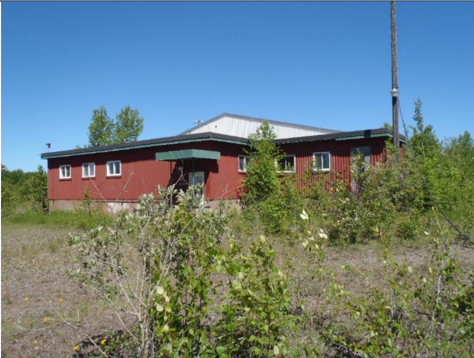
Photo 53: Office part of Office/Warehouse building. Facing northwest.
