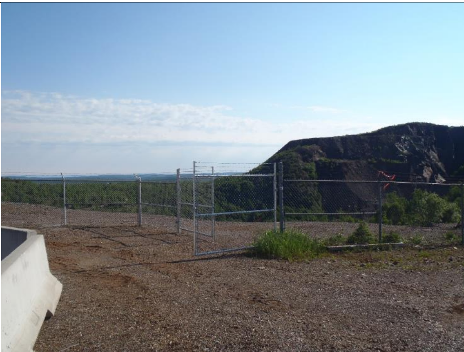
Photo 42: Fence around mine openings. New gate added to accommodate access to drain. Facing north.
