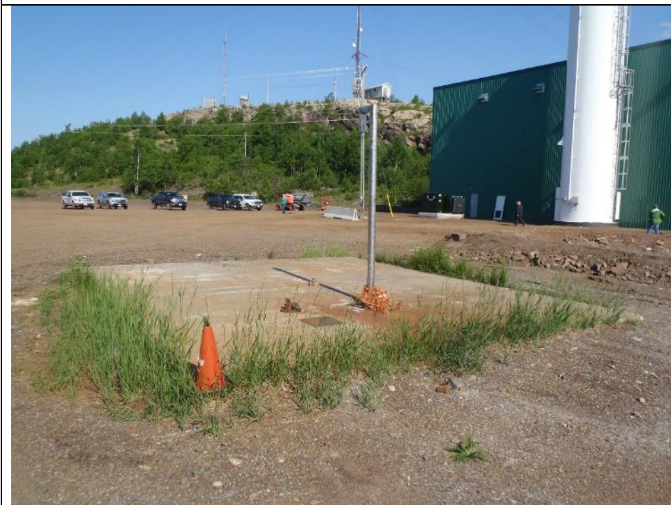
Photo 2: Shaft No. 5 with new water treatment plant in background. Facing northwest.
