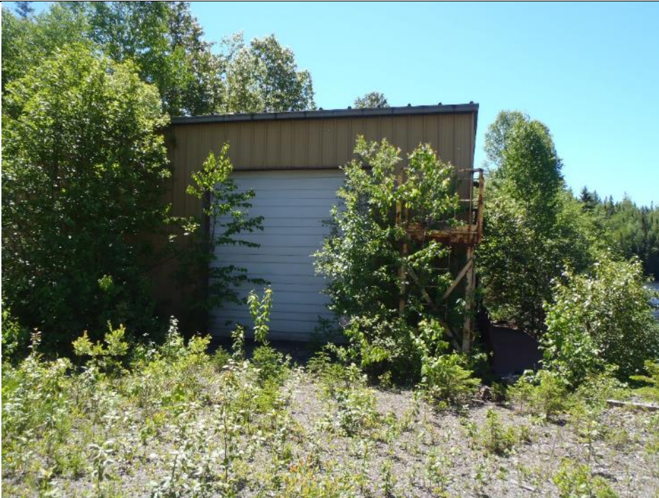
Photo 49: Magpie River Pump house. Facing southeast.
