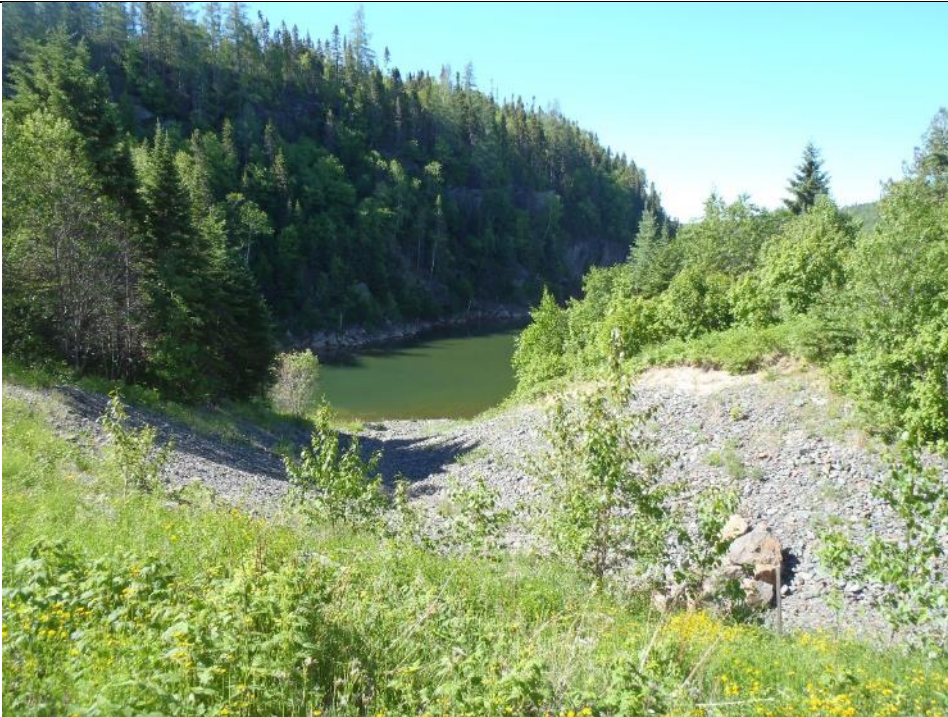
Photo 17: Upper Dam Spillway. Facing south.
