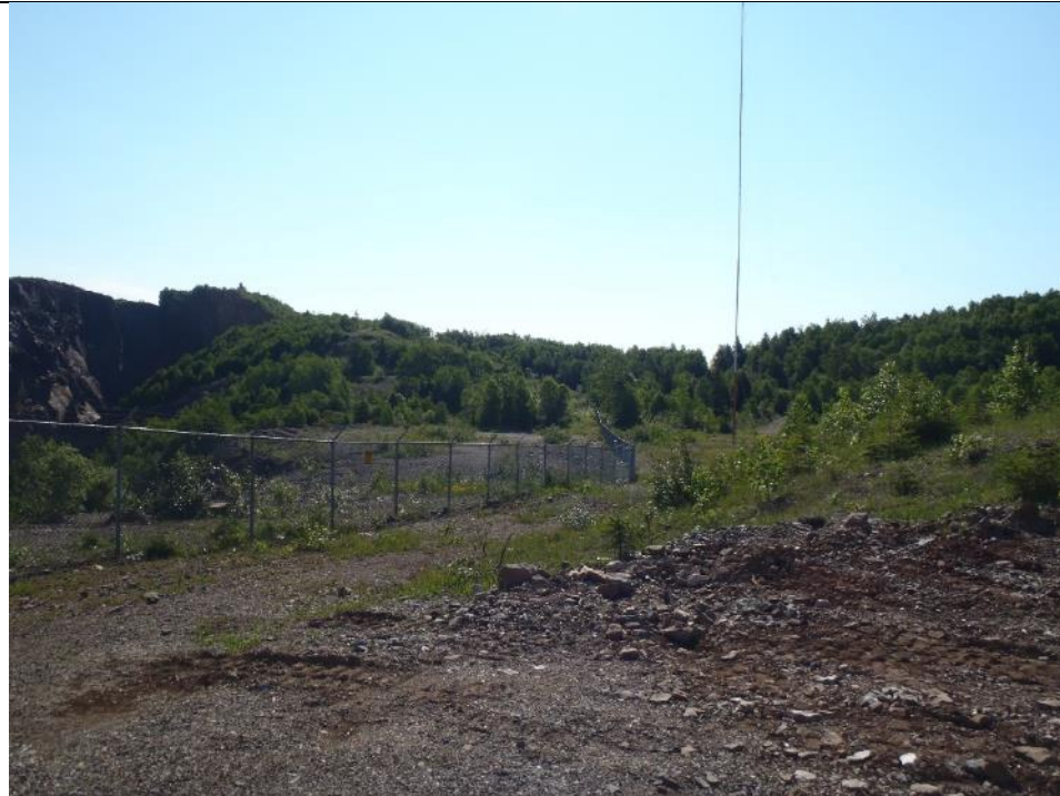
Photo 43 : Fencing around surface openings on mine site in good condition. Facing east.
