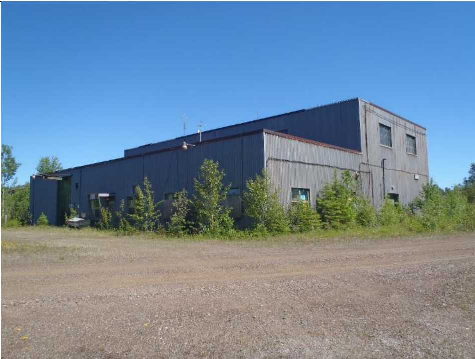
Photo 47: Machine shop showing boarded windows. Facing northwest.
