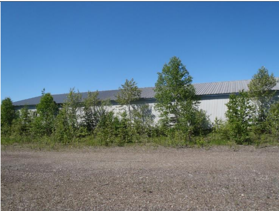
Photo 54: Warehouse part of Office/Warehouse building. Facing southwest.
