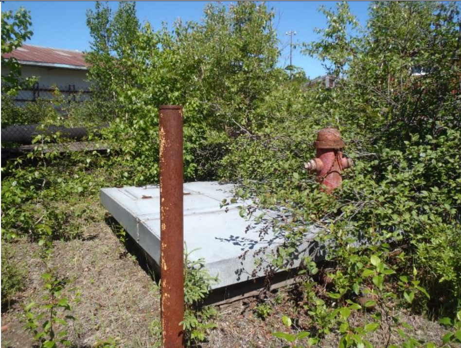
Photo 45: Fire Hydrant Pipe access. Facing northwest.
