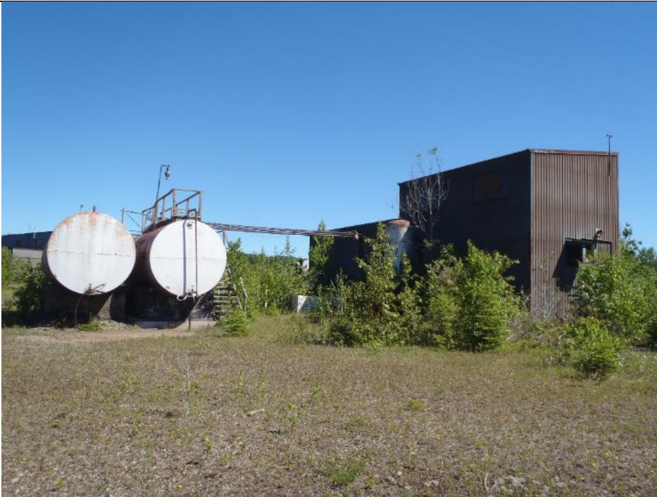
Photo 39: Compressor/Boiler House and oil tanks. Facing north.
