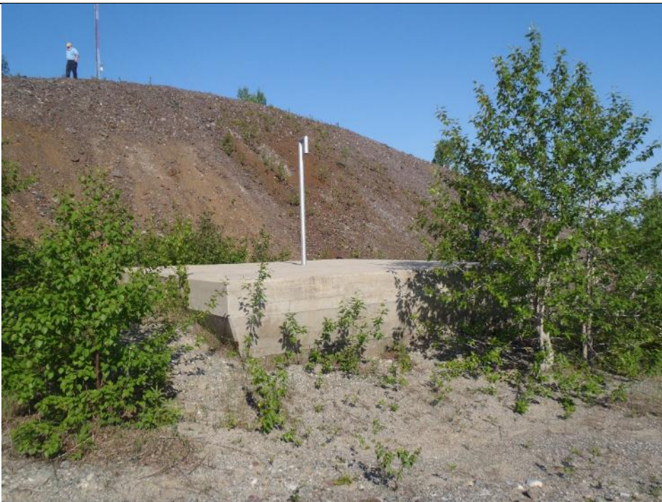
Photo 4: H-222 Exhaust Raise within fenced area. Facing west.
