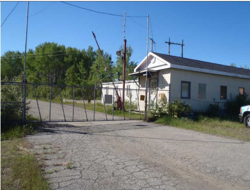
Photo 46: Gate house and gate to Sinter Plant site. Facing south.
