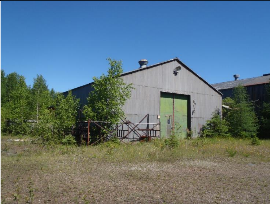
Photo 57: Pipe Shop, front. Facing northwest.
