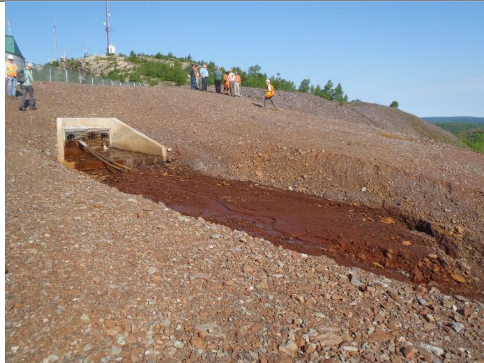
Photo 29: Drain from clarifier to Boyer Lake. Facing west.
