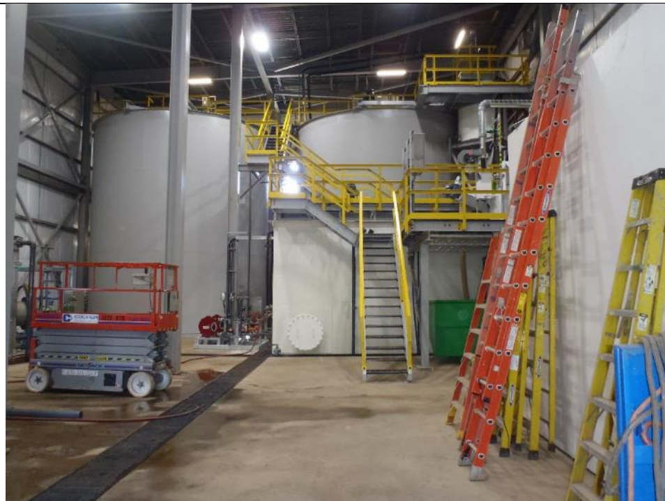
Photo 68: Water Treatment Plant interior. Facing north.
