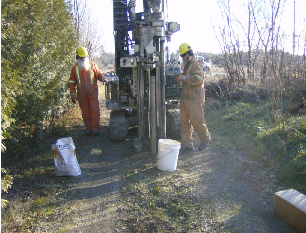
Photo 1 – Site of BH-14
