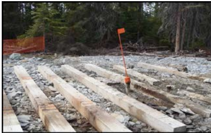
Photo 10: Drill casing with cap and flag to mark it.
