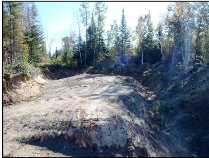
Photo 2: Stripped area greater than 100 square metres stripped, not yet washed.
