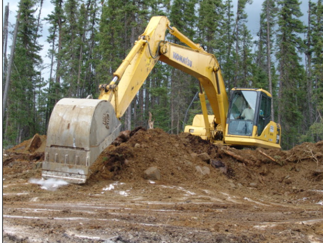
Photo 3: Backhoe being used to strip overburden.
