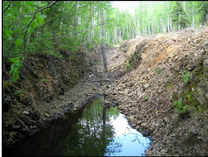
Photo 7: Example of a linear trench in bedrock greater than 3 cubic metres.
