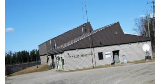
Water Treatment Plant - Geraldton
