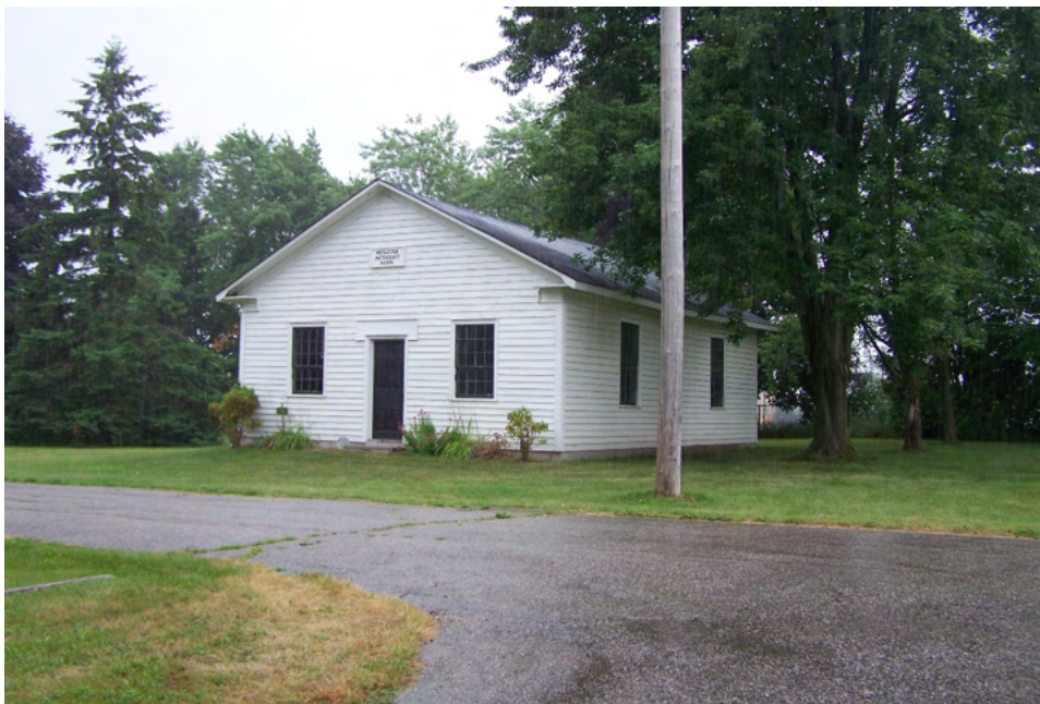
Figure 26. Victoria Square Wesleyan Methodist Church in Markham is a modest 165-year-old wooden frame building which served as a place of worship until 1880, when it was replaced by a larger brick Gothic Revival Church. The building was moved off site and converted to a blacksmith's shop. In 2003, the Victoria Square United Church rallied to purchase the vacant and badly damaged structure. The original wooden chapel was moved back to the church property and lovingly restored (Image courtesy of the Town of Markham).
