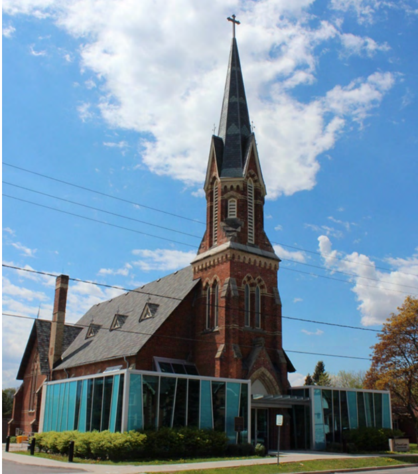
Figure 27. The former St. Francis Roman Catholic Church in Ajax has been converted into the St. Francis Centre, a multicultural space and theatre. This is an example of how a heritage place of worship can be adapted to new use to meet the needs of the community (Image courtesy of the City of Ajax).
