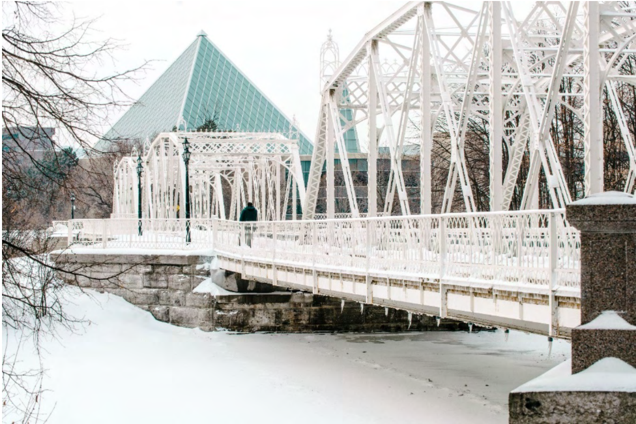
Figure 11. The Minto Bridge spanning the Rideau Canal (Image courtesy of the City of Ottawa).
