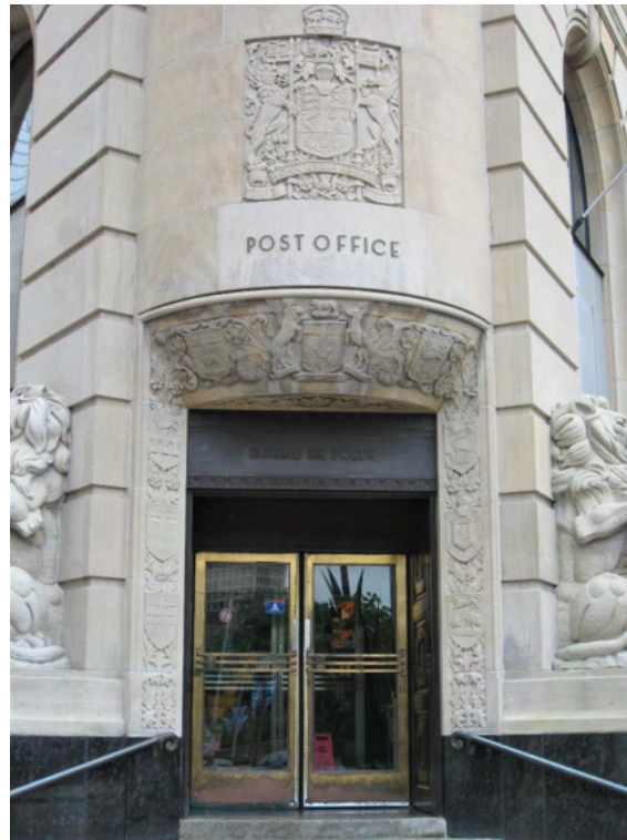
Figure 34. Post office in the Sparks Street Heritage Conservation District (Image courtesy of the City of Ottawa)
