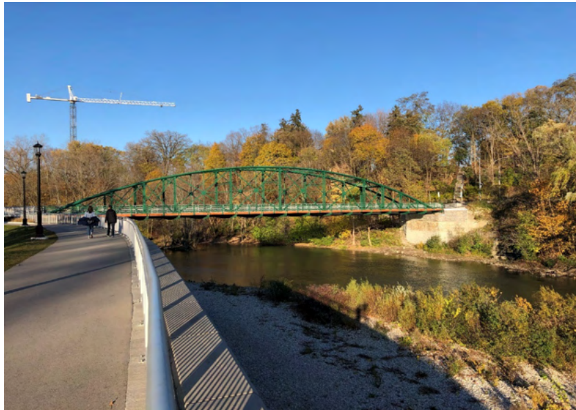
Figure 35. Blackfriars Bridge - 1875 wrought iron bowstring arch bridge underwent a major rehabilitation in 2017-2018 (Image courtesy of the City of London).
