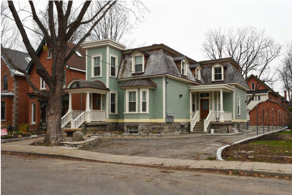
Figure 39. The Simard House (1884) was restored using original materials to help maintain the properties integrity as a rare example of a Second Empire style. Five apartments were able to be added to the structure without compromising the properties integrity of the property's heritage attributes (Image courtesy of the city of Ottawa).
