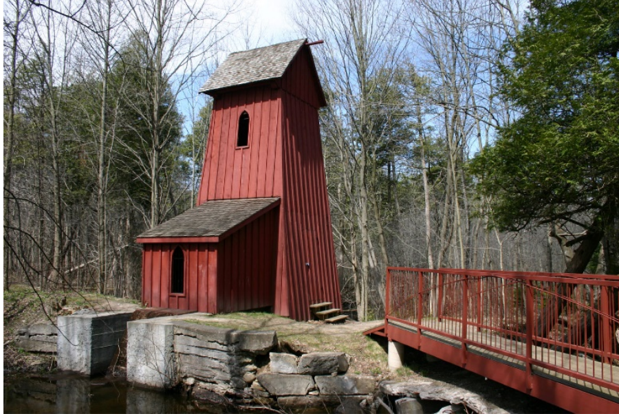
Figure 20. Sheave Tower (MHSTCI)
