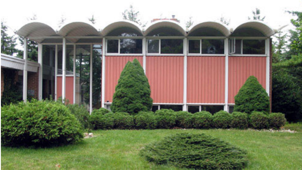
Figure 6. The Pagani House, built in 1961 and designed by architect Richard Pagani as his own home, is one of the best examples in Guelph of modern design (Image courtesy of Frank Hochtchenbach).
