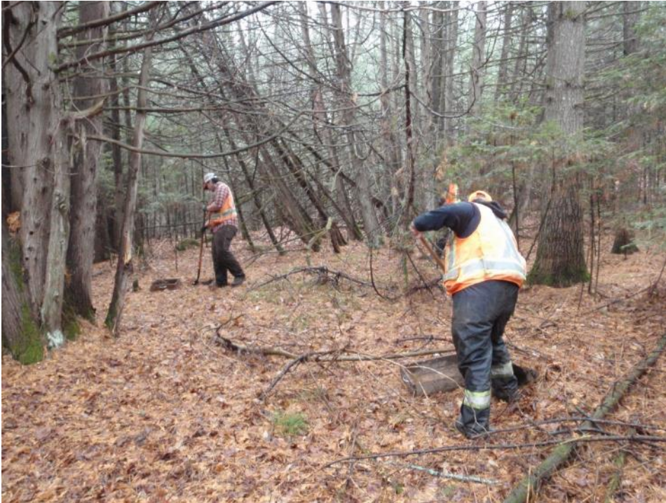
Image 17: Test pitting, facing south.
