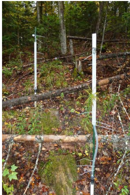
Photograph No. 16 - Manometers - MW4 - Oct-9-14
