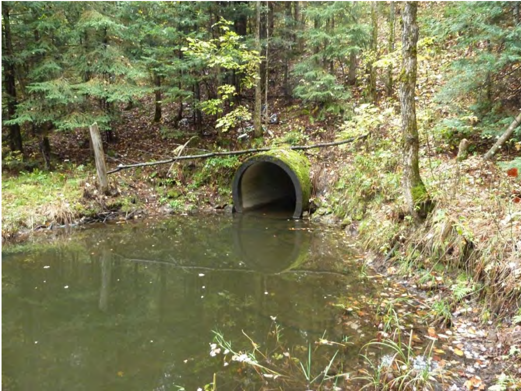
Photograph No. 13 - North Stream - upstream culvert beneath rail trail
