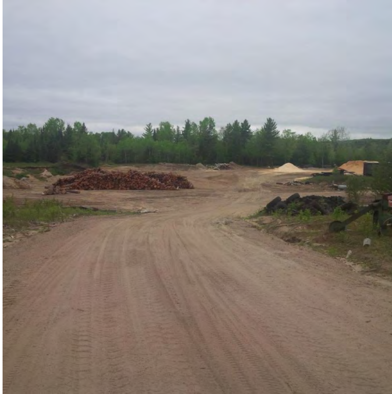
Photograph No. 1 – Existing Pit - License No. 624804 - looking north into pit from the Site
