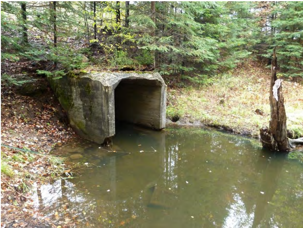
Photograph No. 14 - North Stream - downstream culvert beneath highway
