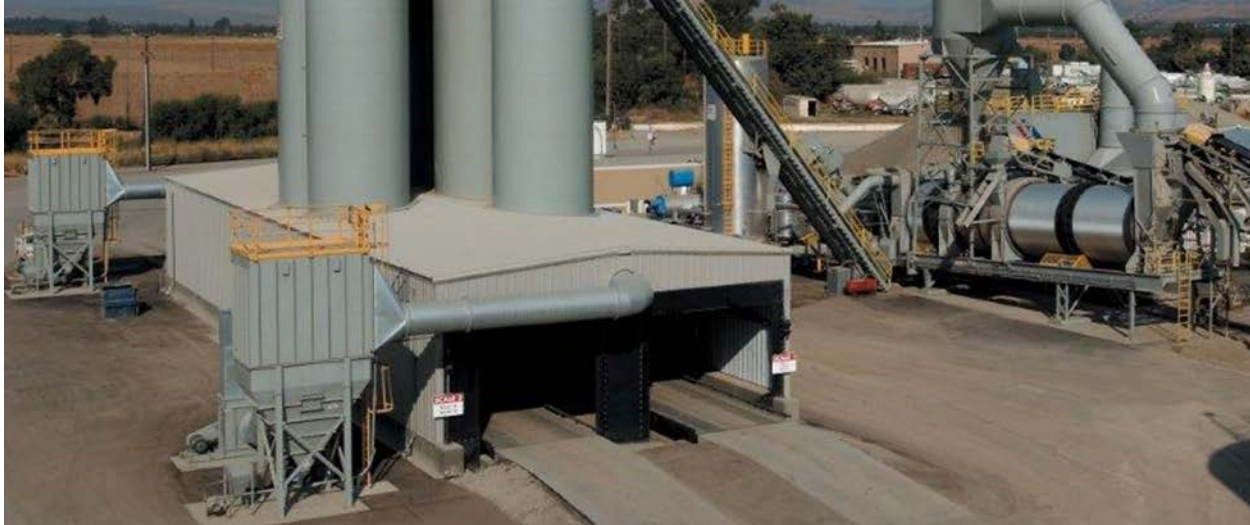
Figure 3 Example of a vapour recovery system which includes enclosure of the loadout point.
